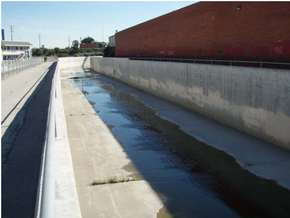
Figure A-2-6 - Downstream of Site 30_VERSEP. Taken on November 4, 2010 at 12:00 p.m.
